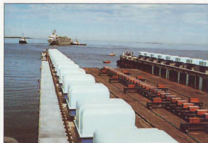
Longitudinal transfer carriage for flatbottom vessels
