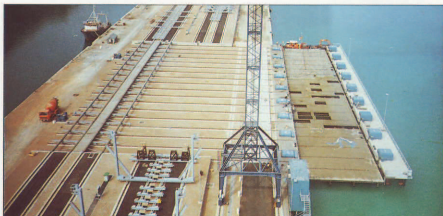
Typical berth and transfer arrangement with lift-dock® at right-hand side
